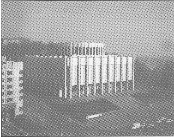
Building housing CUPP office in Kyiv.
